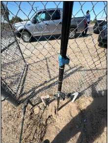
FIGURE 5 - WATER CURB BOX AND HOSE
