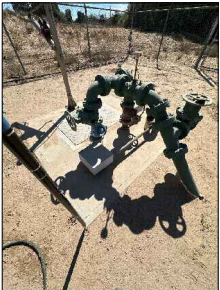
FIGURE 4 - 4" GATE VALVES AND CHECK VALVES
